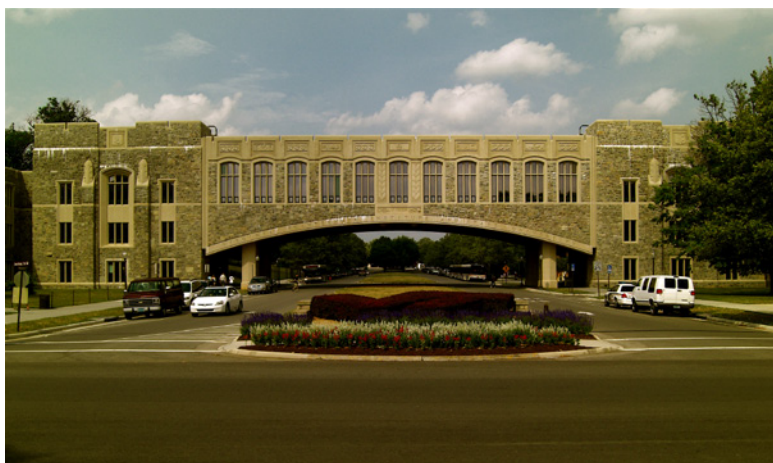
Torgerson Hall Bridge over Alumni Mall on the Virginia Tech campus.
